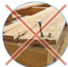
Raised nails great than 1/8" are NOT ALLOWED
